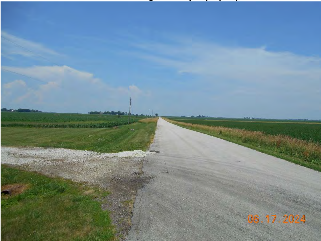
From Subject Property facing N along 1200E.
