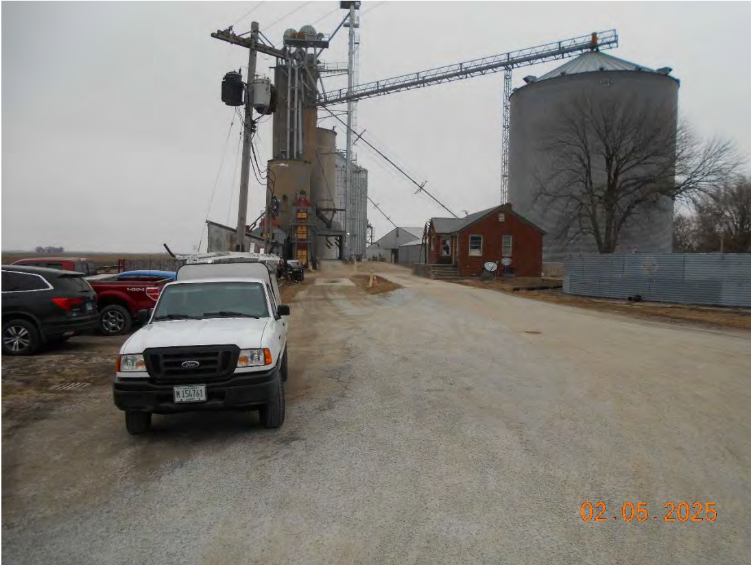
From 3050N looking north at the west entrance of the elevator
