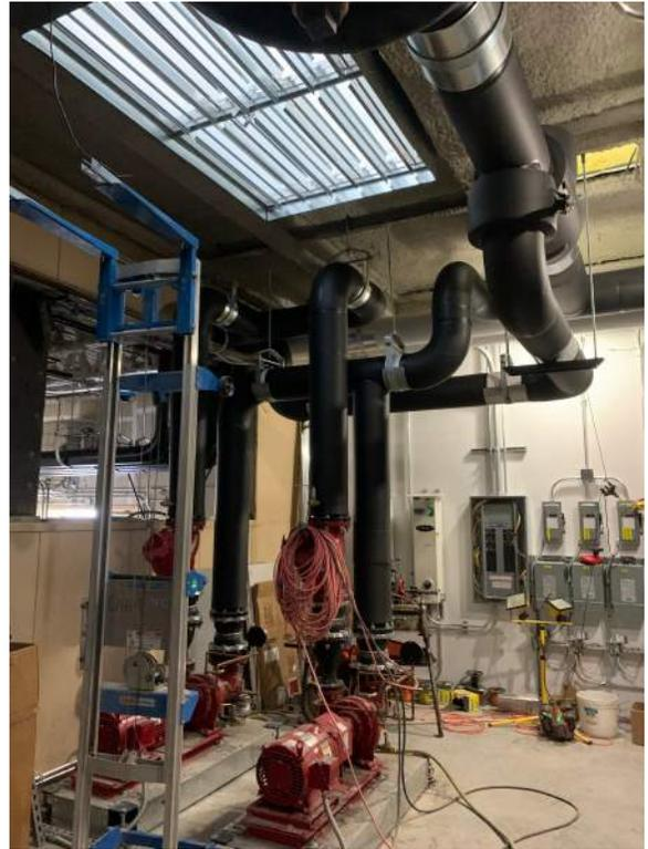
Insulated water pipe connected to pumps.
