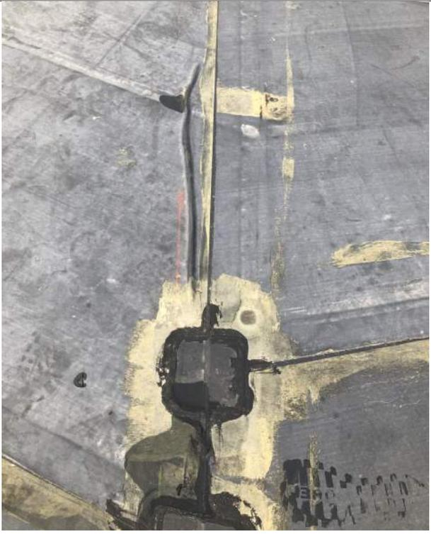
26 Complete base flashings and terminations once RTU is installed.
